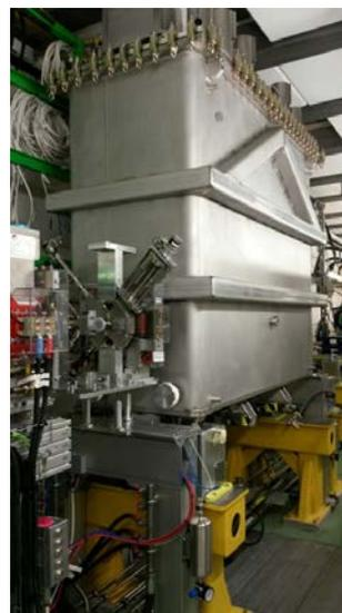
*Fig. 6 Cryomodule 2 being connected to its services in the HIE-ISOLDE tunnel*
