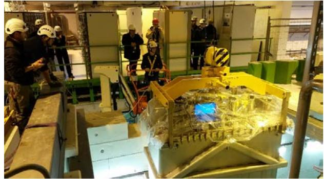
*Fig. 5 Dismounting cryomodule 1 in the HIE shielding tunnel for retro fitting of the RF couplers in SM18*
